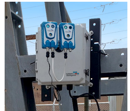
Figure 1 – IM500 thermal plus visual sensor module can be installed close to high power.
