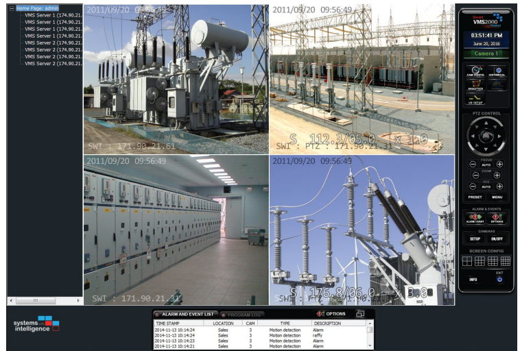
VMS2000 Client Main Screen
