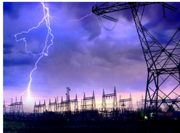
Figure 3. Lightning Protection: Making a Wise Investment for your Smart Grid, Buildings.com
